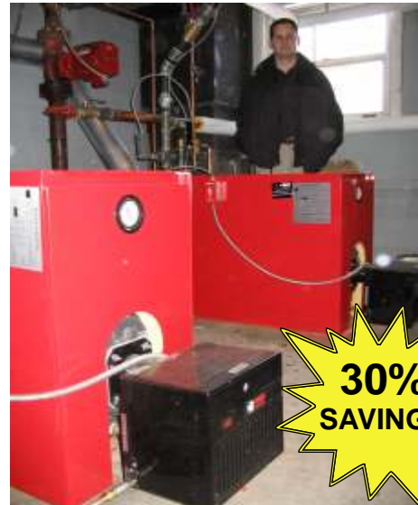
Bill LeRoy of LeRoy's Heating showing the two BIASI B-10, 8 section oil fired boilers equipped with Riello F10 Oil Burners installed at Millidge House in Saint John, NB.
